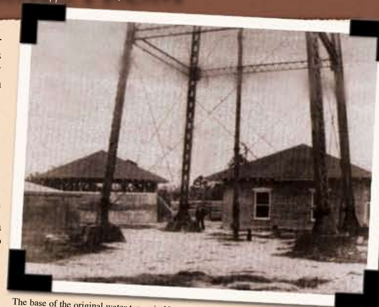
The base of the original water tower in New Smyrna Beach, also located at the Smith St. site. The back building quite possibly held pump equipment and a well. The bricks, used as foundations in this 1927 picture, are still sometimes discovered on the property.
