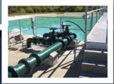
The backwash water recovery basin and pumping equipment, Glencoe Water Treatment Plant
